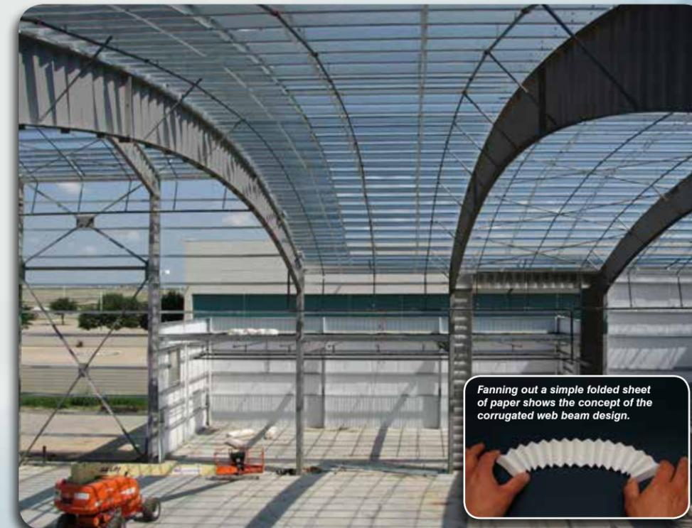
Fanning out a simple folded sheet of paper shows the concept of the corrugated web beam design.
