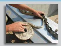
Mastic between all panel joints and foam sealer at the base provide a protective barrier against moisture and wind.
