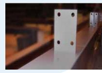
Behlen clips are pre-welded for a better fit and reduced erection cost and time.
